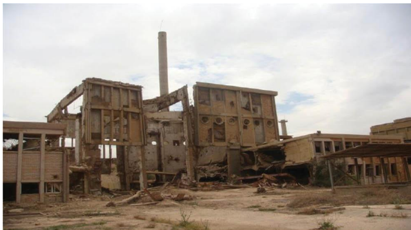
Figure 2 – The destroyed Nuclear Reactor at Al-Tuwaitha nuclear research site [25]
