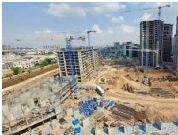
Figure 3 – Construction activities in Erbil (Moveit Magazine, June 2020)
